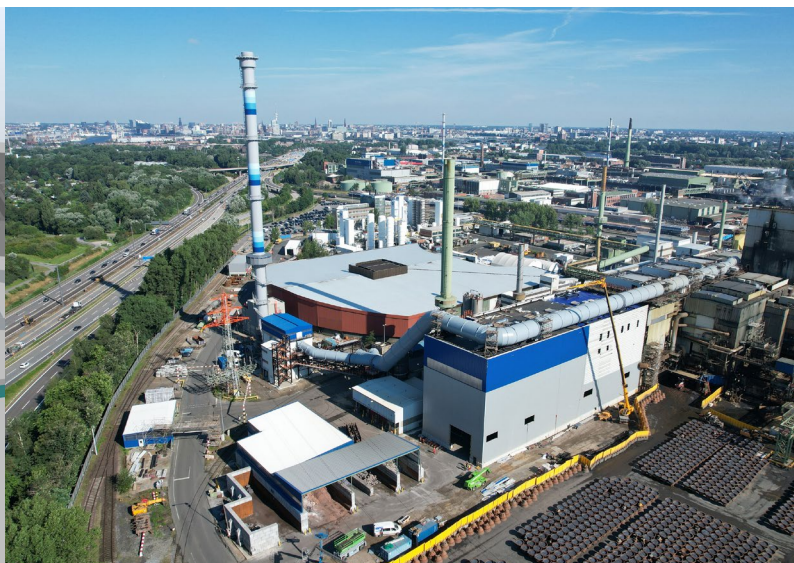
RDE expansion stage 1 at the Hamburg site
